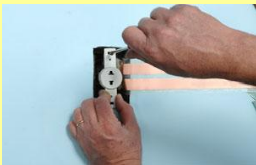
Reinstalar a tomada original
